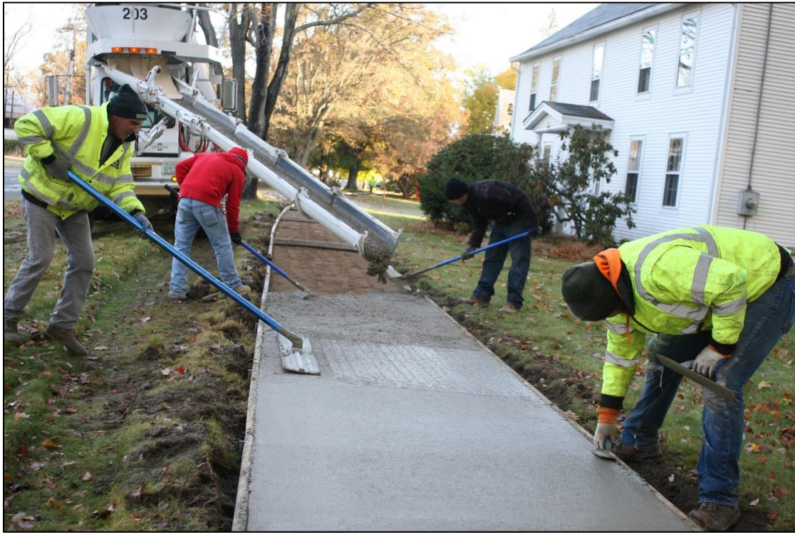
Hatfield DPW installing sidewalks on Main Street.
