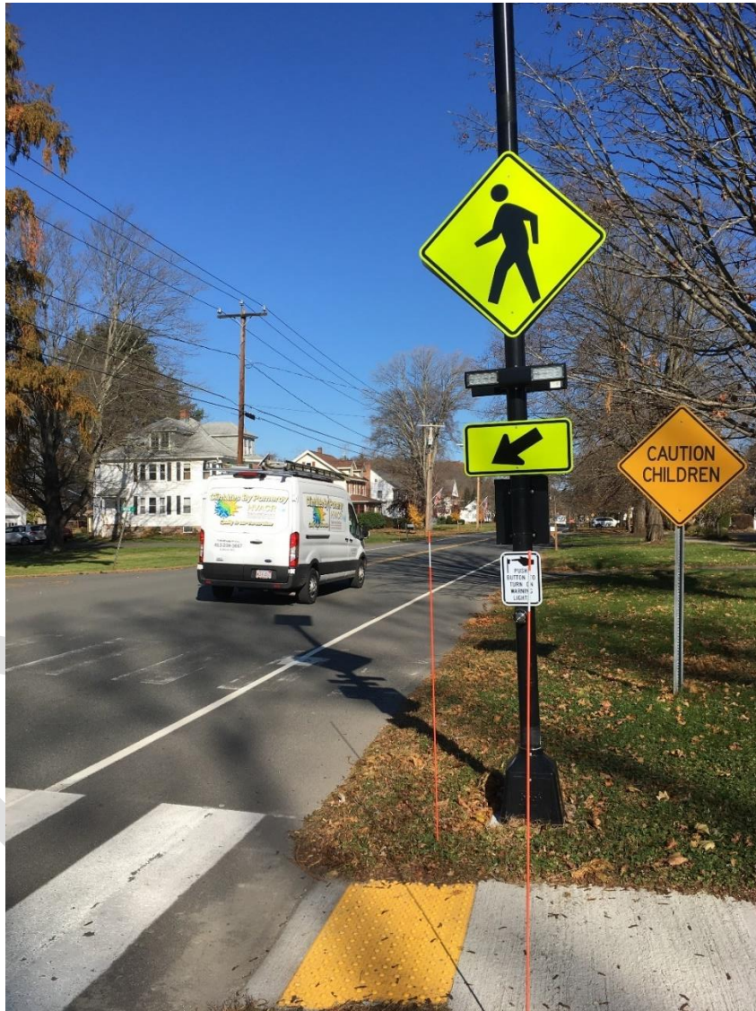
Hatfield DPW installed Rectangular Rapid Flashing Beacons pedestrian actuated signals on the Main Street intersection with North Street in 2023.
